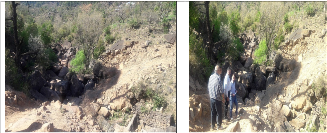
Link road Mansar to Sourap in PIU Udhampur physically inspected on 17.03.2018
