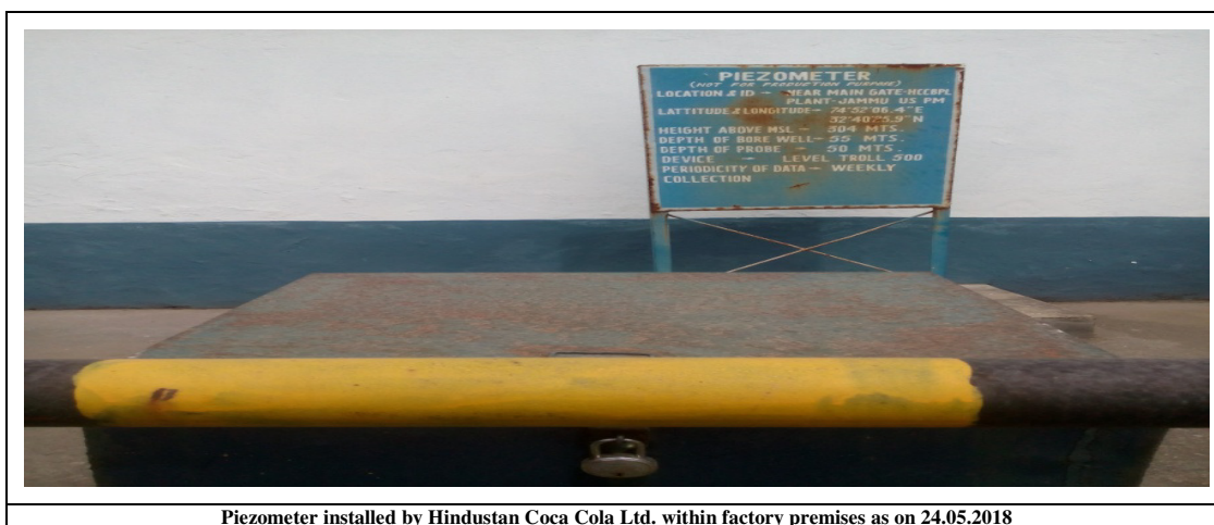
Piezometer installed by Hindustan Coca Cola Ltd. within factory premises as on 24.05.2018
