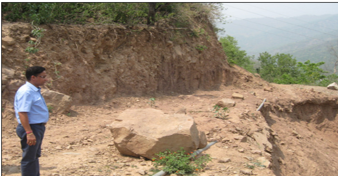
Damaged portion of Poonda Khul At RD-1900 M
